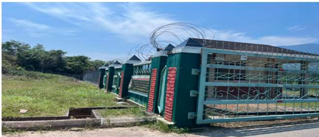
Diagram 1.4 (b): Fence Installed in Front of the Aruk National Border Post (PLBN) Source: Field Study at ICQS Biawak Complex on October 2, 2023
